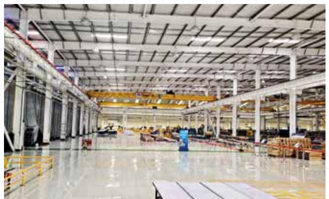
Natural light provided by the SunLite Strip™ daylighting system is one of the features of the interior of the Xi'an facility.
