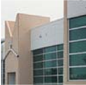
Commercial and Industrial Panels
