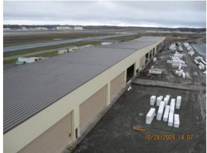
U.S. Air Force Alaska Hangars
